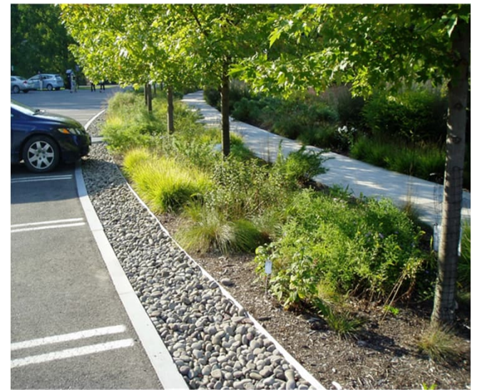
Source: Tompkins County NY (Bioswale)
