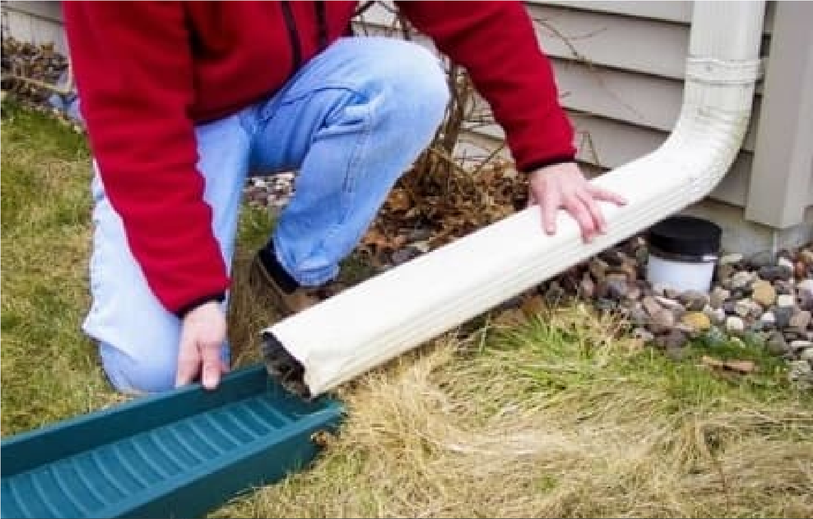
Downspout Disconnect
