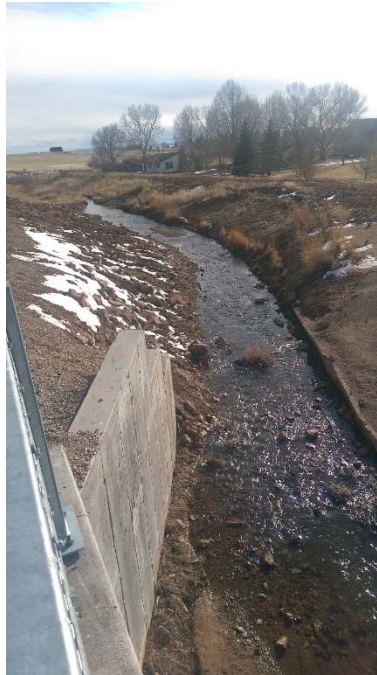
SC290 – 30 th Street Bridge Downstream Left: 0.035, Middle: 0.030, Right: 0.035
