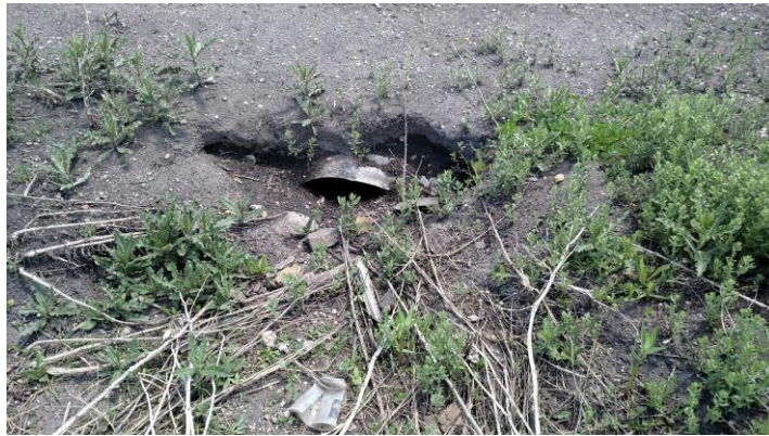
Picture 4: Existing 36-inch Culvert at 1 st and Sanders Street – West End
