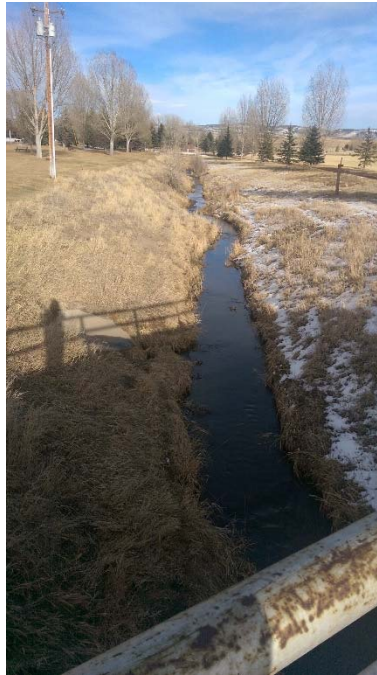
SC275 – Bridge on Corthell Street Upstream Left: 0.035, Middle: 0.030, Right: 0.030
