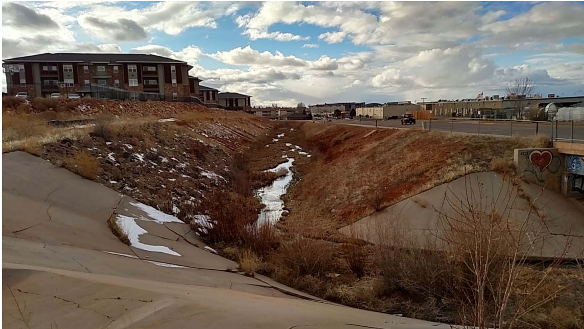
SC295 – 30 th Street Bridge Downstream Left: 0.027, Middle: 0.030, Right: 0.030
