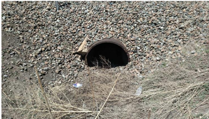
Picture 3: Existing 36-inch Culvert at 1 st and Sanders Street – East End
