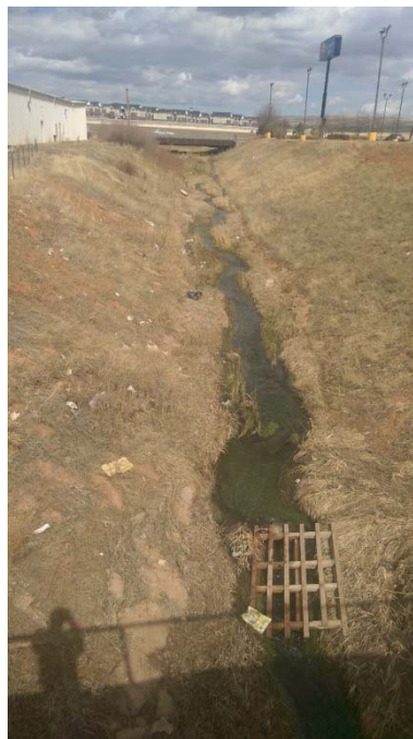
SC297 – 30 th Street Bridge Upstream Left: 0.027, Middle: 0.030, Right: 0.030
