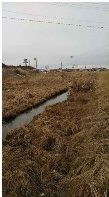
SC210 – Around 5 th Street Downstream Left: 0.035, Middle: 0.040, Right: 0.045
