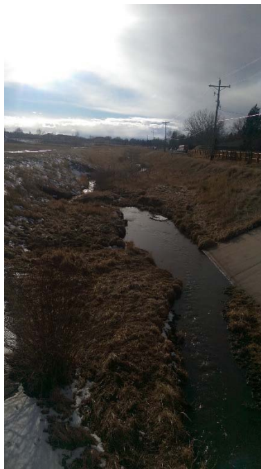
SC265 – Bridge on Corthell Street Downstream Left: 0.035, Middle: 0.030, Right: 0.035
