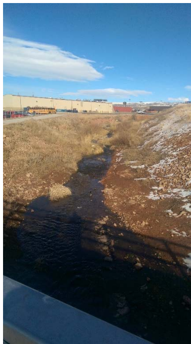
SC295 – 30 th Street Bridge Upstream Left: 0.027, Middle: 0.030, Right: 0.030
