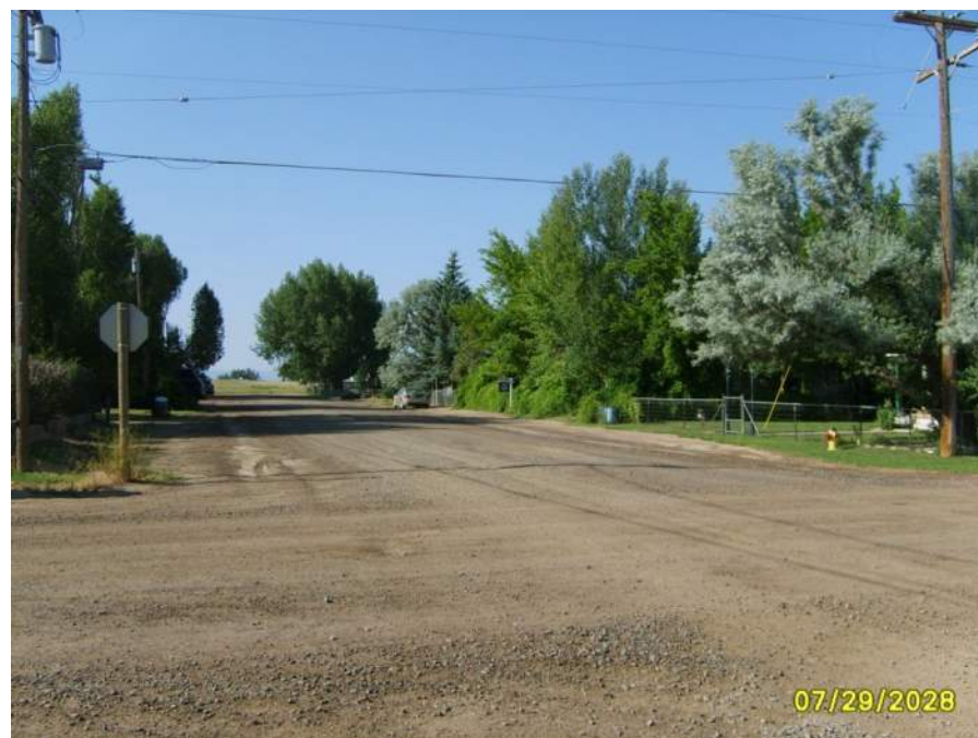
Photo 10: Harrison St. and Grant St.
