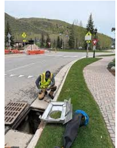
Gutter Bin Installation in Casper WY
