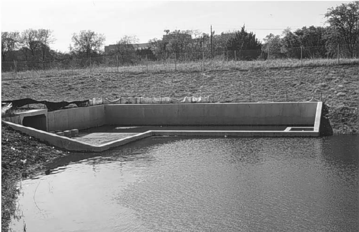
Concrete lined detention pond in Austin, TX
