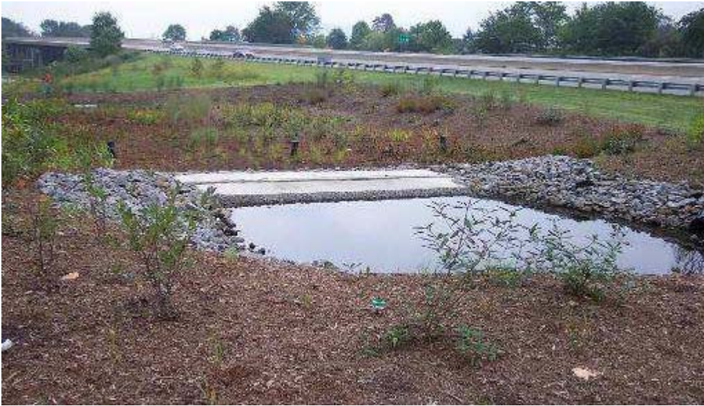
Detention pond (background) with forebay (foreground)
