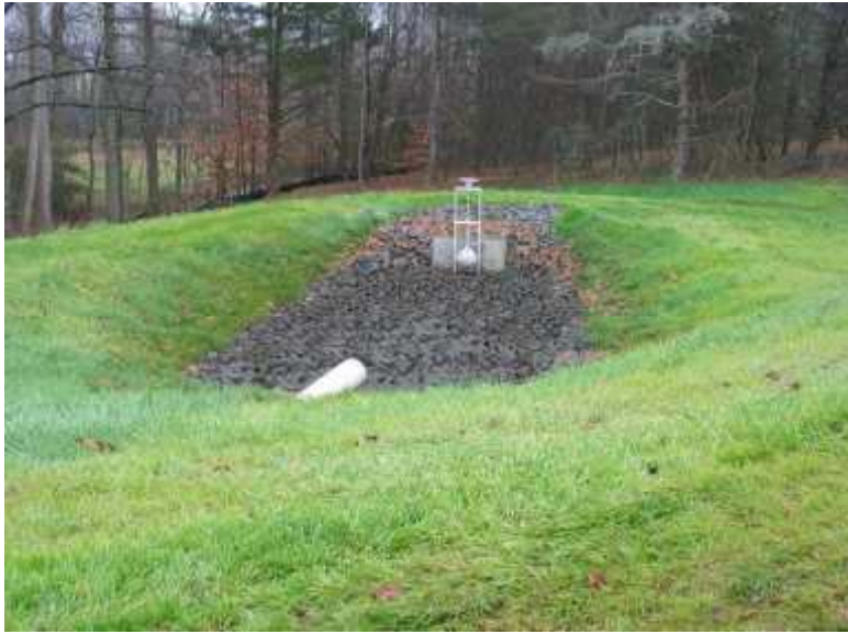
Hazardous Spill Basin
