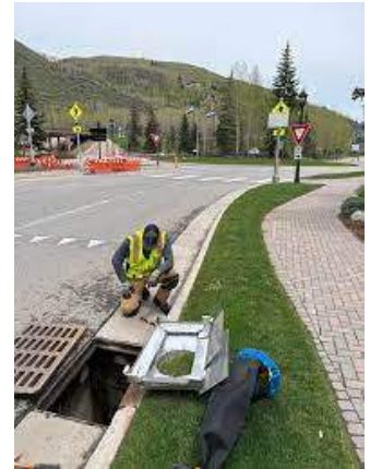
Gutter Bin Installation in Casper WY
