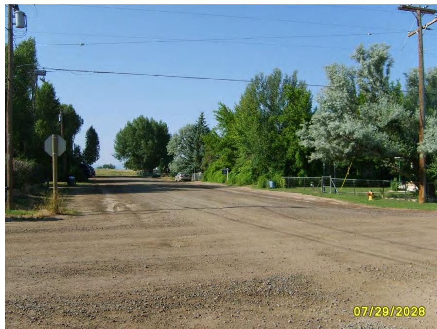
Photo 10: Harrison St. and Grant St.
