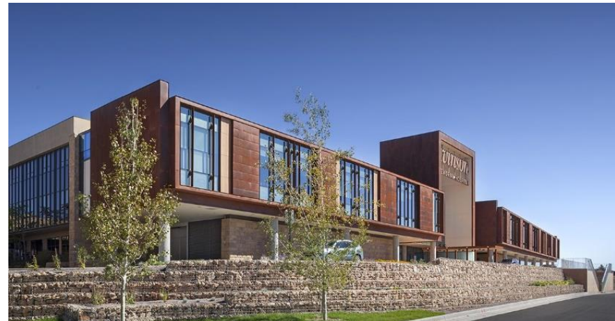
Figure 31: Ivinson Memorial Hospital
