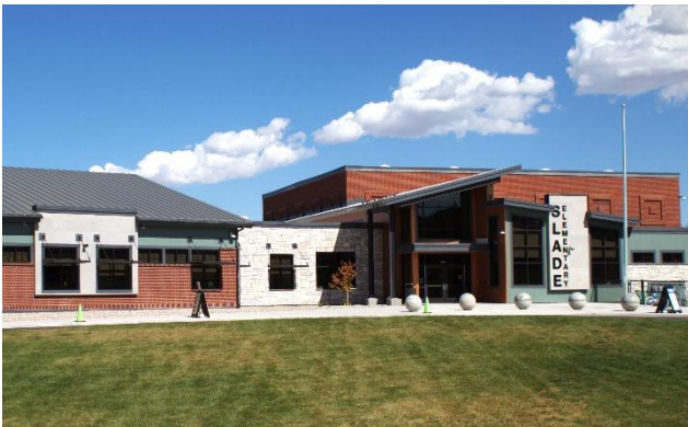
Figure 15: This route serves several k-12 schools, including Slade Elementary, which would facilitate staff commuting to work.
