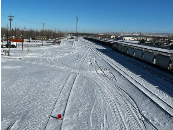
Crossing I-80 and UPRR
