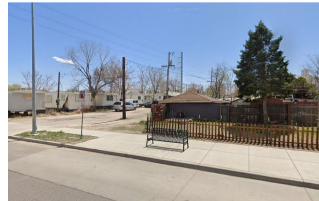
Figure 23: Example of typical new stop amenities: ADA landing pad in front of sidewalk, bench, sign, light from nearby streetlight. Concrete bus pad not included in this plan. No shelter at most stops.
