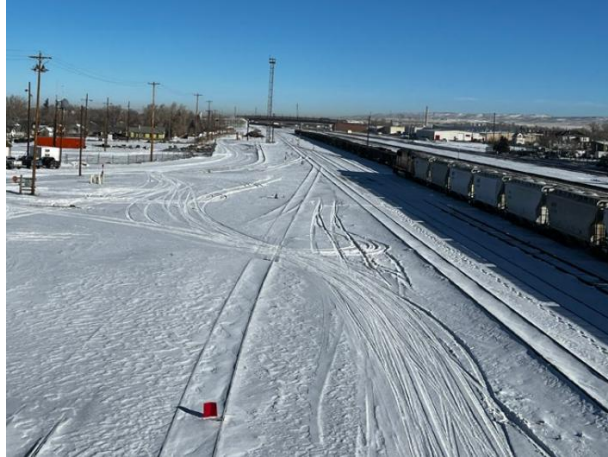
Crossing I-80 and UPRR
